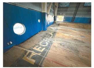
The new ovm's wooden floor was buckled from heat and water damage.
