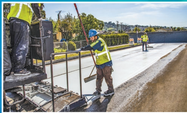
Crews apply the cool pavement.
