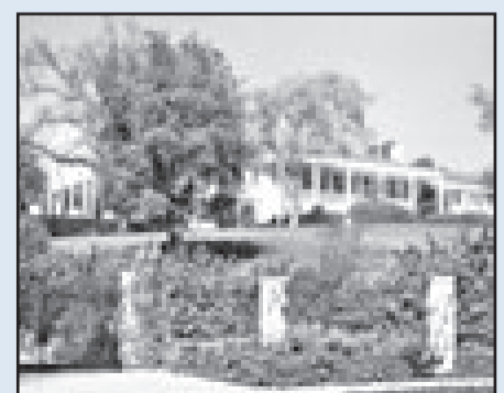
A private residence designed by Paul R. Williams.
