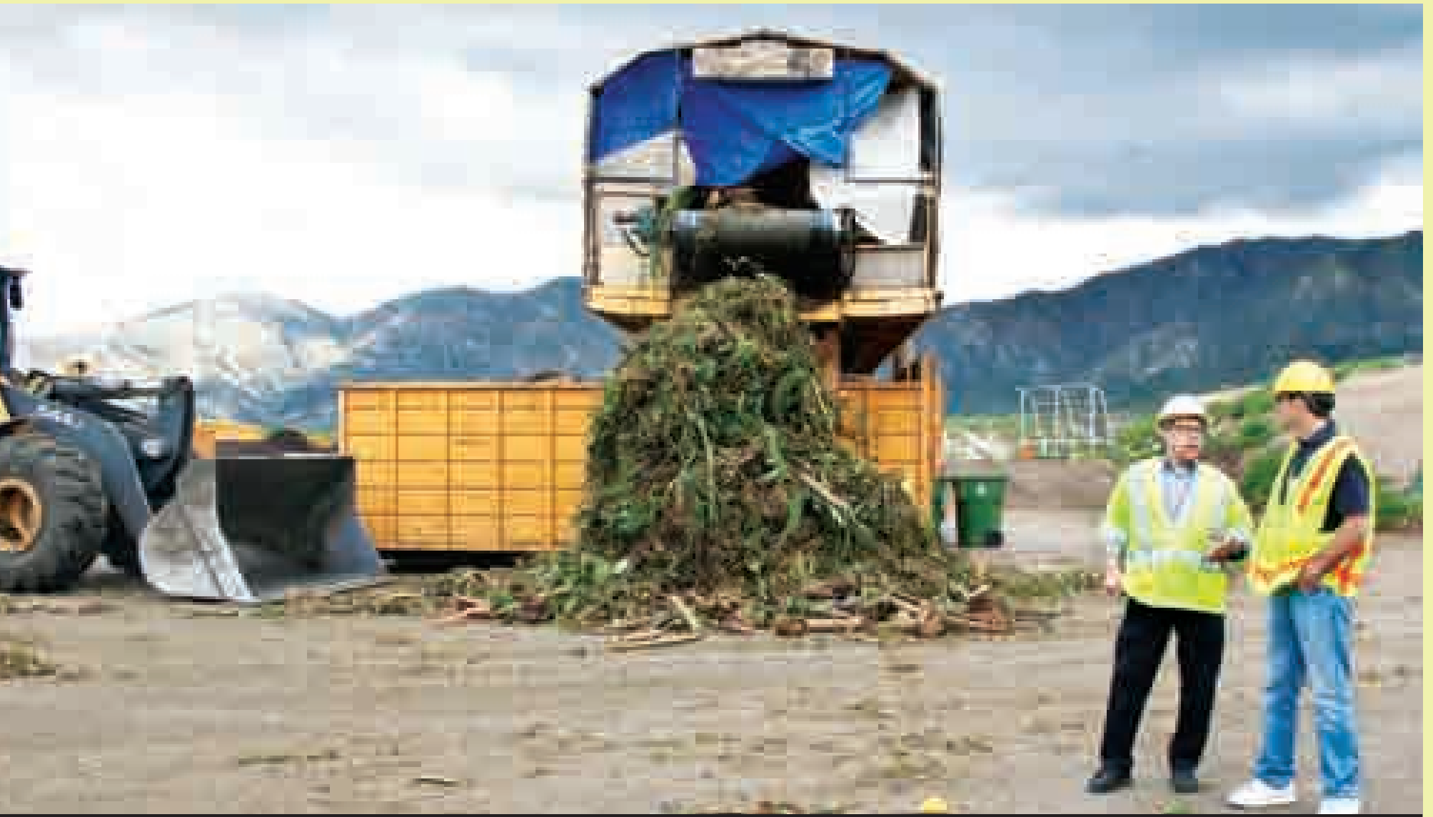
The Lopez Canyon mulch processing facility.
