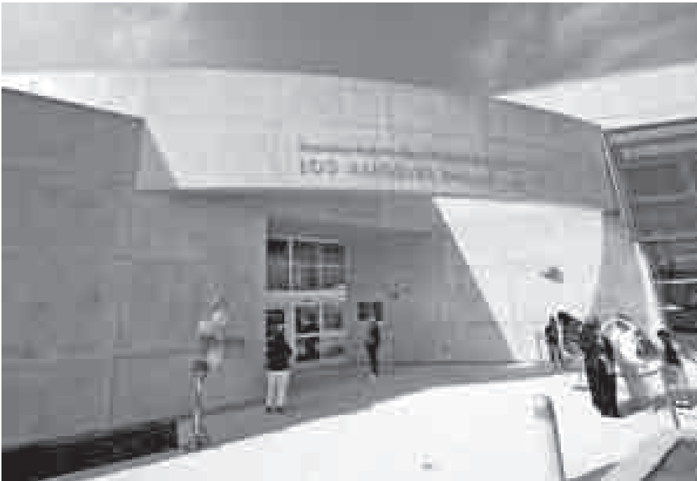
The new Exposition Park – Dr. Mary McLeod Bethune Regional Branch Library, the “greenest” building in the Eighth Council District.
