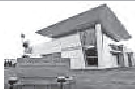
The new Harbor Gateway Branch Library.
