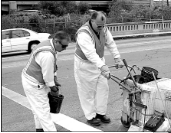
Thermoplastic Operators striping the street.
