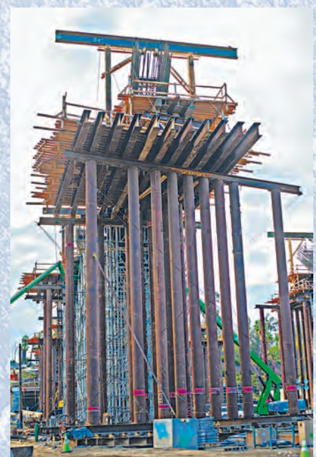
The new Sixth Street Viaduct under construction.
