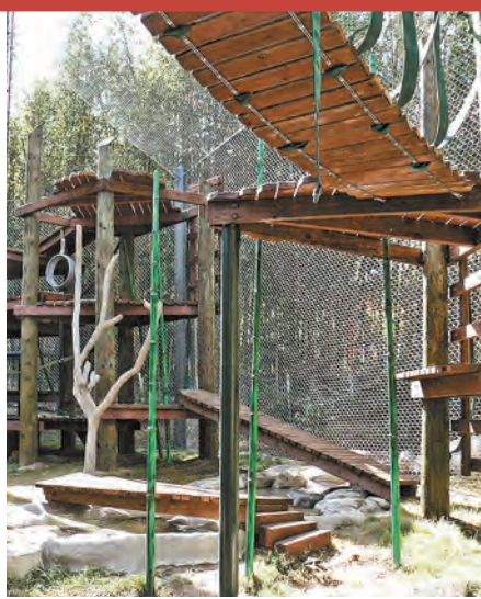
Red Ape Rain Forest structure renovations
