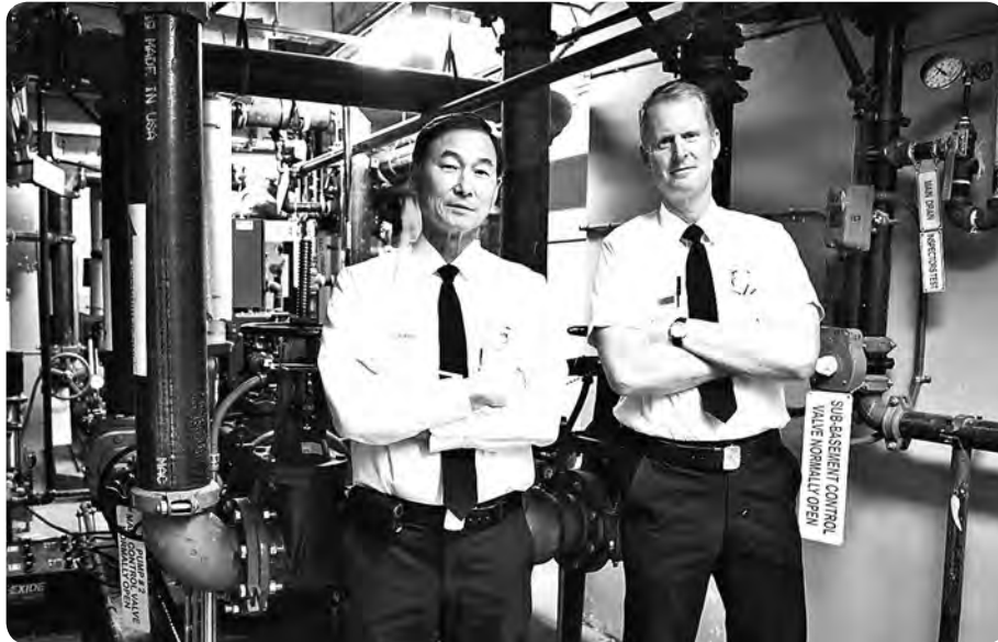
Lloyd Fukuda, Research Unit Inspector I, and Mark Chase, Fire Inspector II for New Construction, in the pump room below the SB Spring Building.
