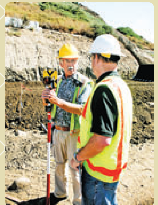
ABOVE: Rick Allen, Field Engineering Aide, 25 years of City service, explains the surveying portion of the Potrero Canyon Slope Stabilization Project to Alive! editor John Burnes.
