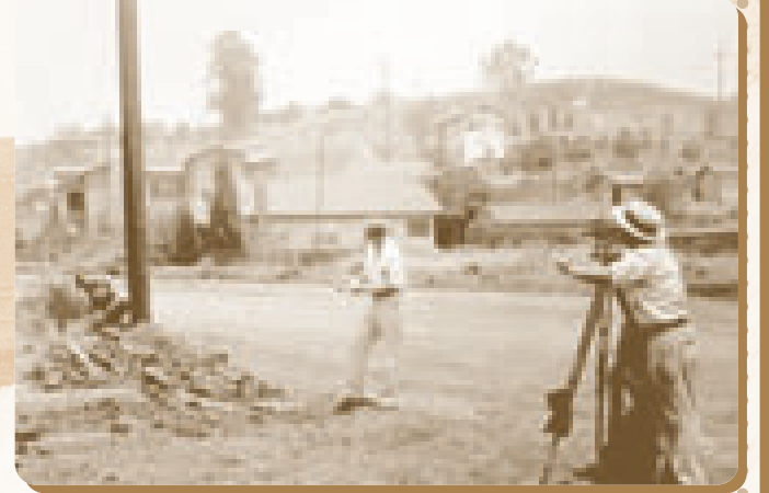
City survey crew providing staking for new curbs.
