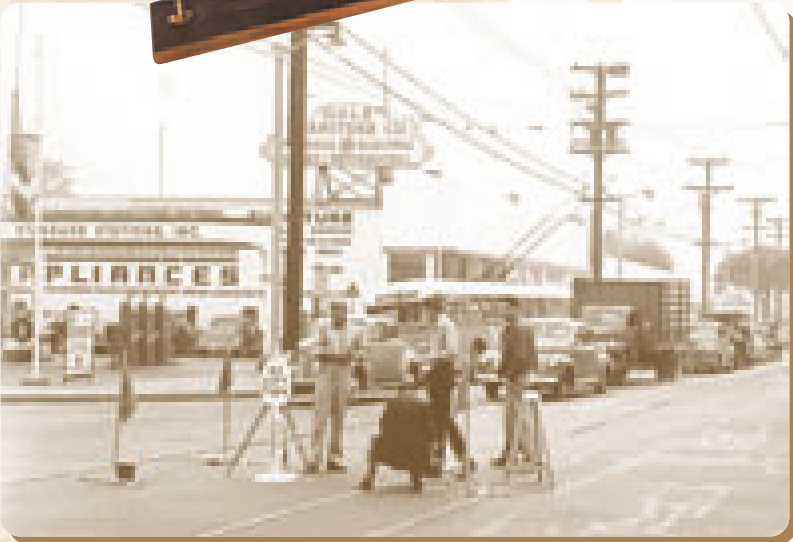
City survey crew establishing the center line intersection of the streets. A cast iron monument cap, still in use today, is seen at the left and is anchoring the "homemade" traffic safety flag.
