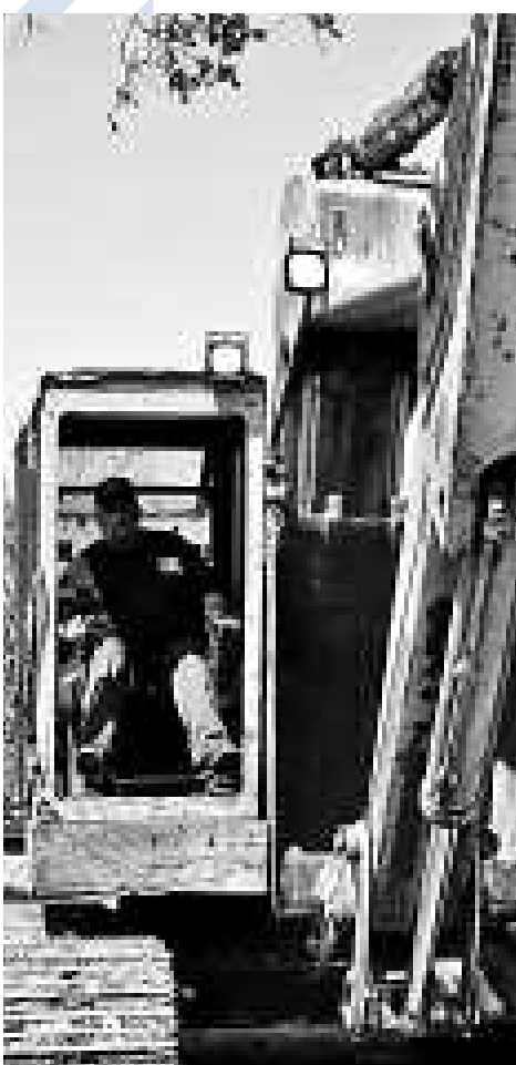
USAR Heavy Rigging Specialist Mike Fennessey, DWP, uses an excavator.
