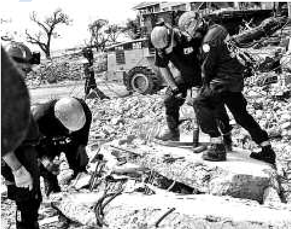
City USAR Team Members "core" a hole for search cam access.
