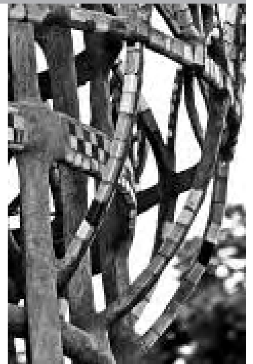
Immigrant Simon Rodia spent 33 years building the Towers, which are both large-scale and highly detailed.
